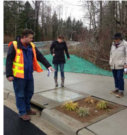
Figure 7. Modular Wetland Stormwater Filter Systems, James Street.
