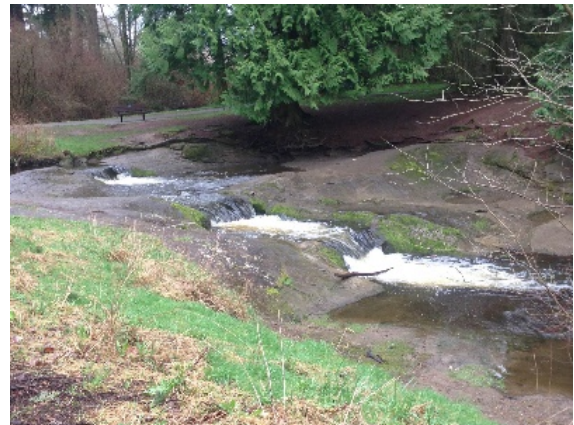
Figure 8. Cornwall Park Notched Fish Way.
