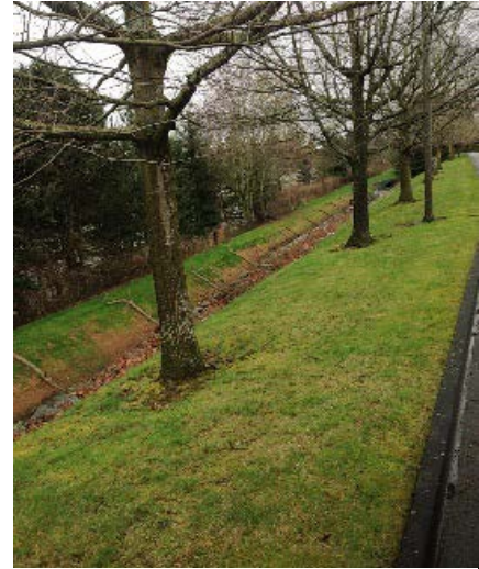
Figure 5. Grassy Bioswales Along I-5, Adjacent to Bellis-Fair Mall.
