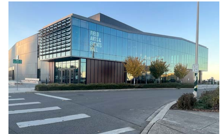
Figure 34. The Field Arts and Events Hall, part of the Port Angeles Waterfront Center just east of Valley Creek.
