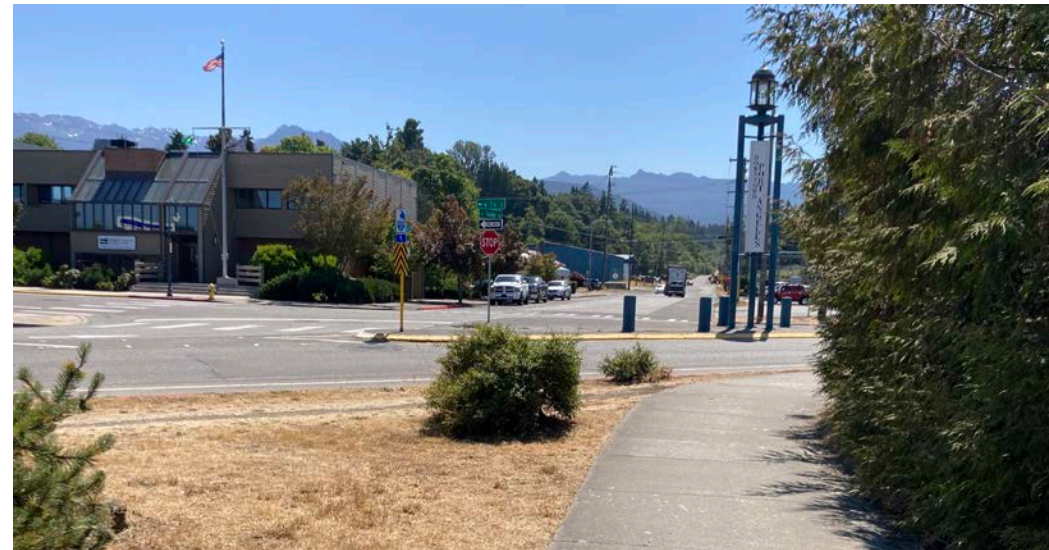
Figure 60. View looking south up South Valley Street where Valley Creek flows through culverts under the roadway
