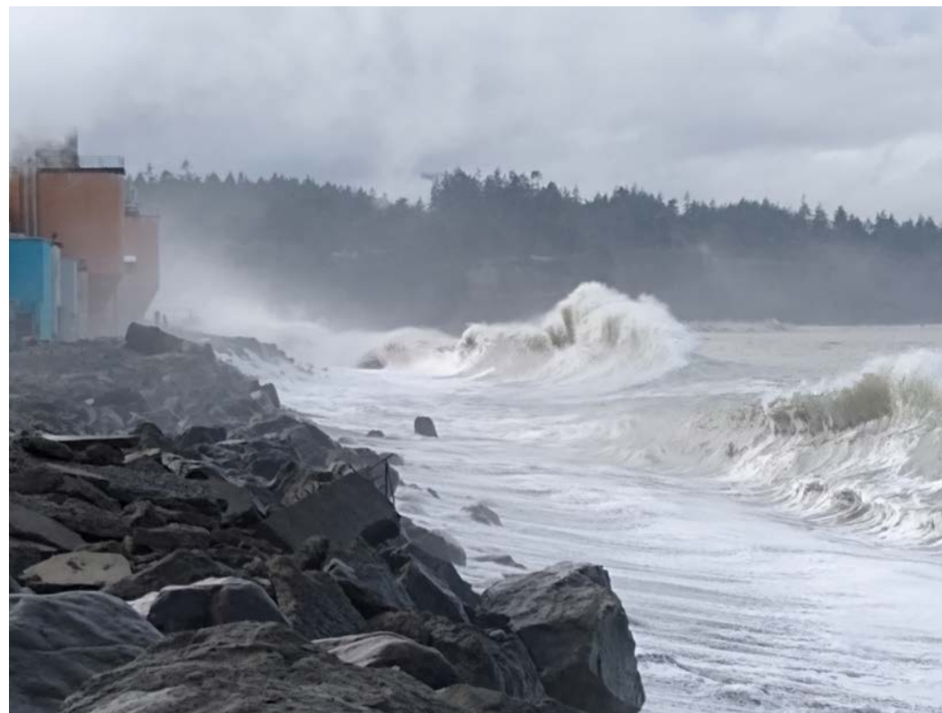
Figure 90. King Tides coinciding with winter storm waves, part of a widespread and damaging event along Washington's shorelines in Jan 2021. Image credit Ian Miller, Washington Sea Grant
