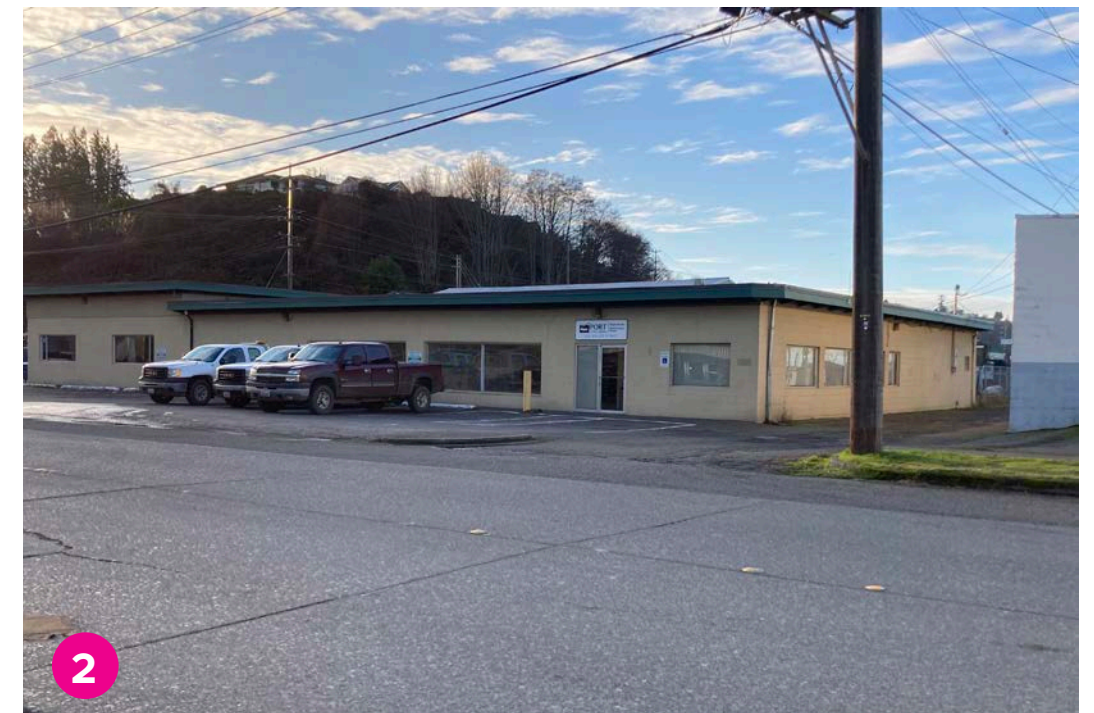
Figure 40. Port of Port Angeles Maintenance Annex building
