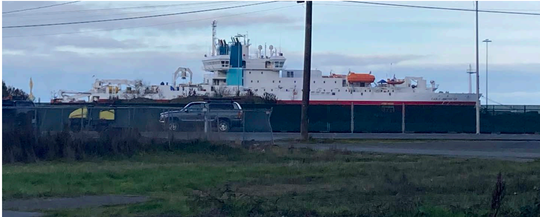
Figure 44. Site of the planned Marine Trade Center in the background, zoned Heavy Industrial
