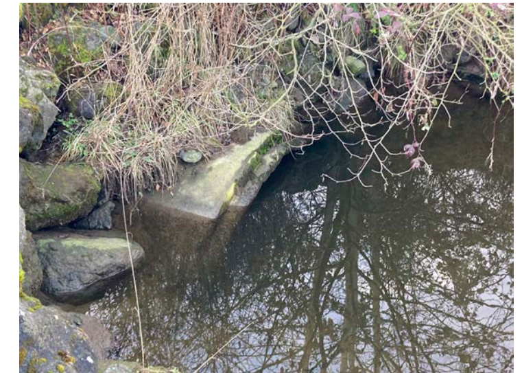
Figure 61. Submerged outlet of Valley Creek culvert
