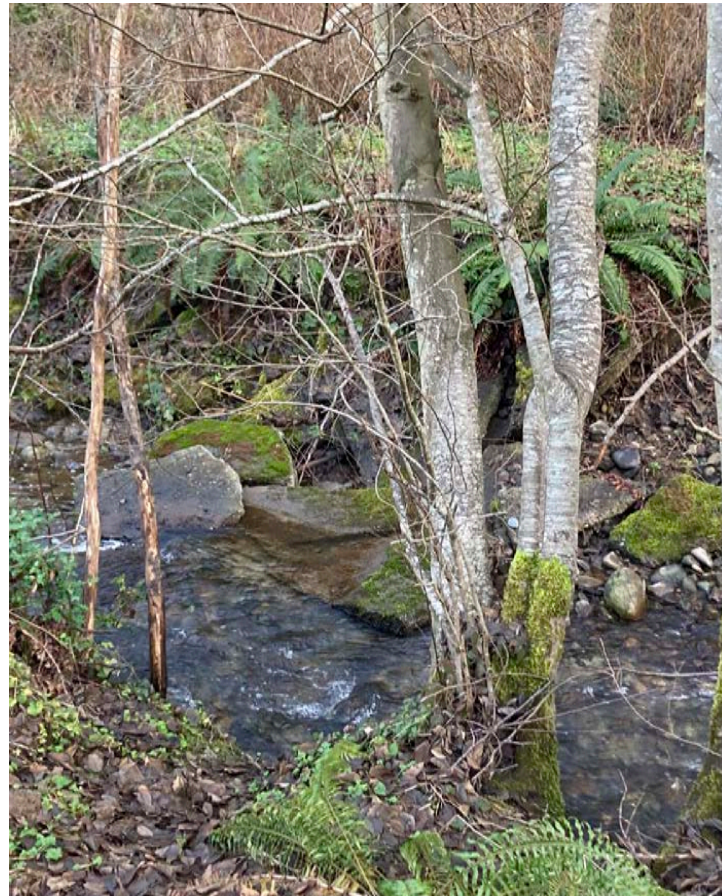
Figure 79. Bank armoring along Valley Creek that is falling into the water
