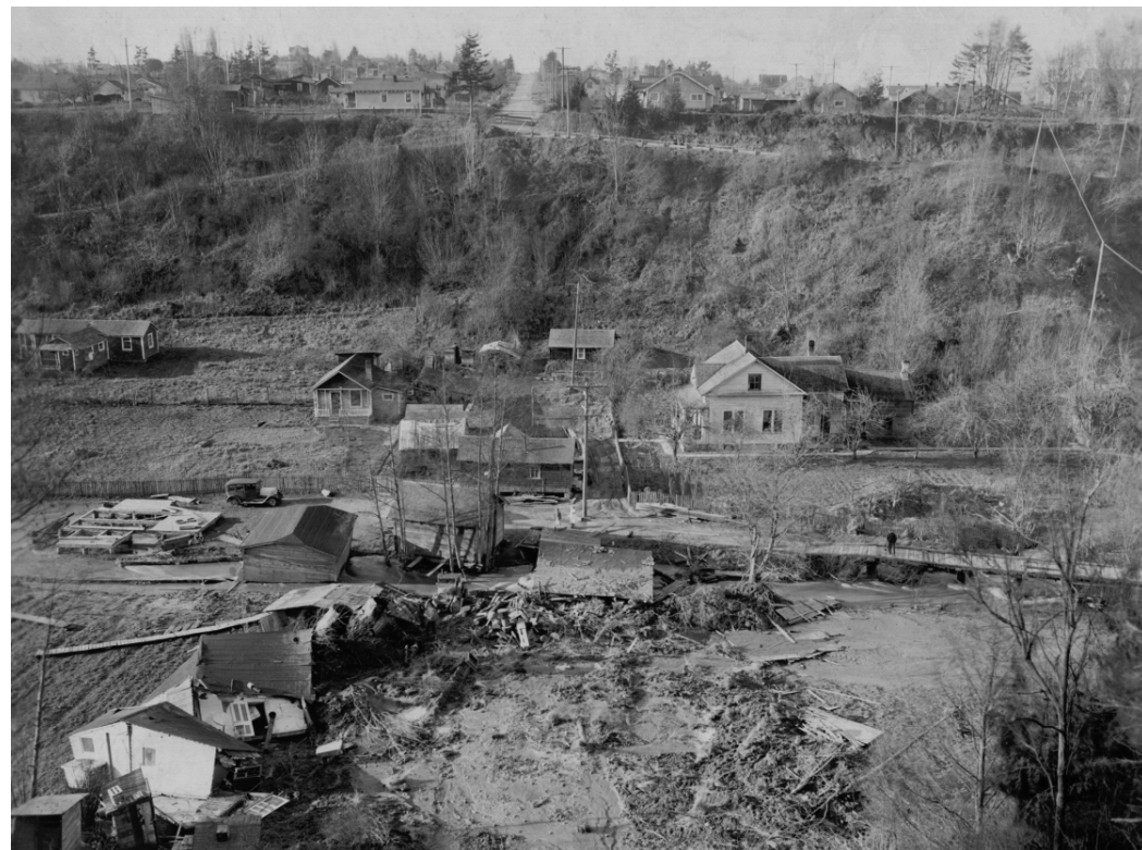
Figure 27. Valley Creek Customs House flood site. Source: Photo courtesy of North Olympic History Center, 2023
